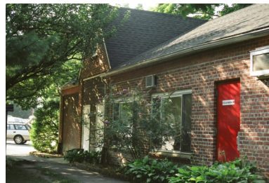
Gillespie Center & Hoskins Place Emergency Shelter for Single Men and Women
